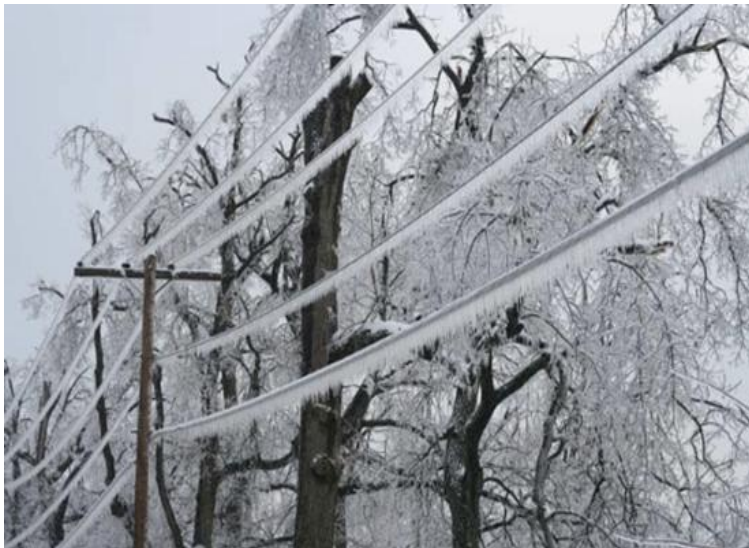
Figure 46 Ice Covered Powerlines
